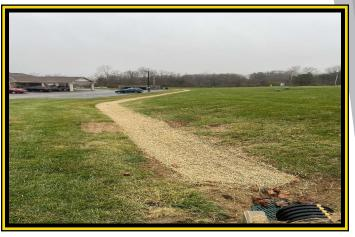
Finally, crews replaced a 36" x 40' culvert pipe on East Pekin by Township Line Road.
