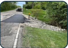
Toward the end of the month, crews began work on the pickleball court extension. They provided drainage tile to the site by digging two feet deep and installing 300 feet of drainage. Crews also applied 135 tons of rock and hired a company to pave the court.
