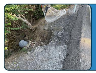
On August 26<sup>th</sup>, crews began a culvert pipe extension repair on Bunnell Hill Road. Heavy spring rains eroded the soil, causing the six-foot extension pipe to drop. As work began, crews noted the damage continued beneath the roadway, creating a potential hazard. Crews instituted an emergency road closure for the repairs, which required a 36-inch, 20-foot pipe, concrete, four tons of asphalt, and 48 tons of rock.
