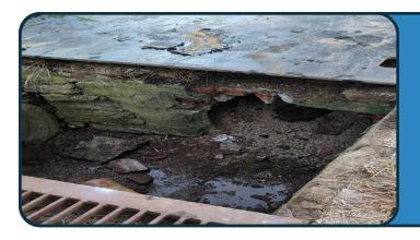
On August 22<sup>nd</sup>, crews changed a 30-inch, 30-foot-long culvert pipe at the intersection of Utica Road, using ten tons of asphalt and 24 tons of rock. This project required rebuilding a handmade catch basin wall around the pipe, using materials stored in-house.
