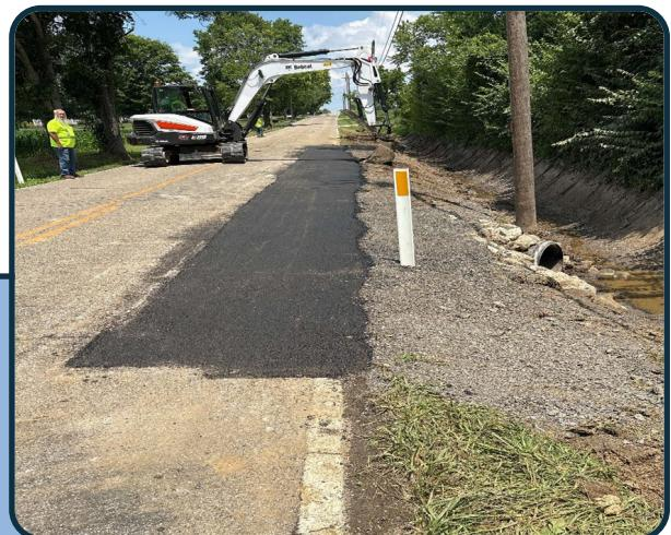
In July, crews ditched the area in the 5200 block of Hathaway Road. Crews moved the ditch by three feet to allow for the addition of a culvert pipe extension. After installation, crews paved the road over the pipe.
