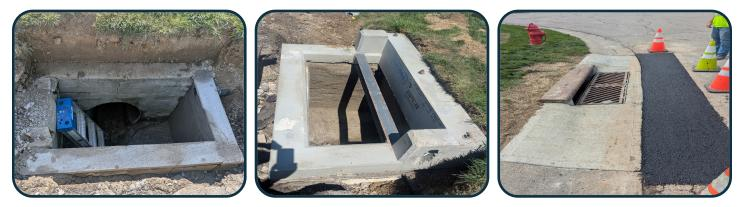
Road Maintenance Crews ended the month repairing a catch basin in Crown Point. The heavy rainfall washed away portions of the catch basin wall, causing the top to collapse six inches into the basin. Crews blocked the walls and fabricated a new top using five yards of concrete and two tons of asphalt.
