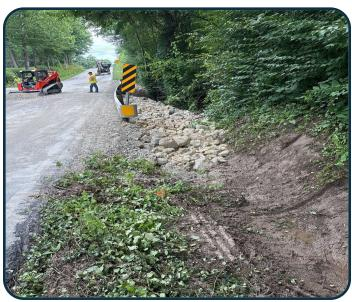
On July 9th, crews ditched the area in the 5200 block of Hathaway Road. Crews moved the ditch by three feet to allow for the addition of a culvert pipe extension. After installation, crews paved the road over the pipe.
