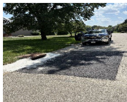
Catch basin repair on Innsbrook Ln
