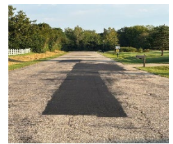
Preparing roads for cape sealing
