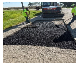
Preparing roads for cape sealing
