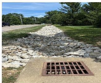
Completed drainage improvements on N Bunnell Hill Rd
