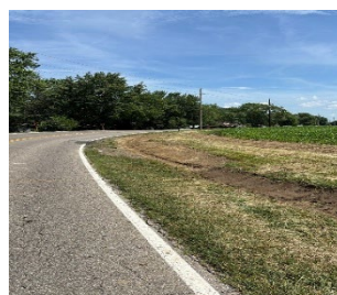
N Bunnell Hill ditch repair
