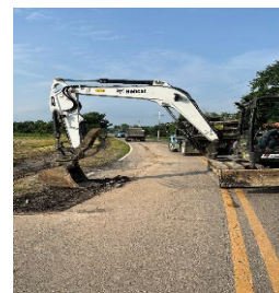
Repaired soft spot in the curve on N Bunnell Hill Rd
