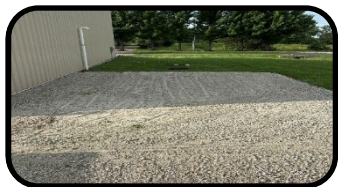
Leveled pads for Fire Station 22 & 23
