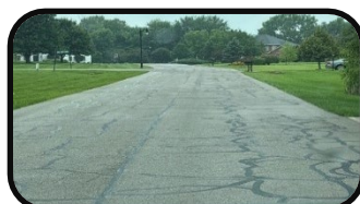
Crack sealing in Cypress Ridge
