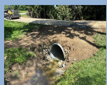
Culvert replacement on West Pekin Rd.
