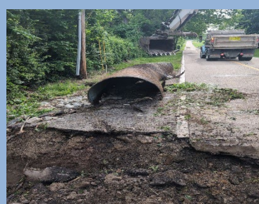
Culvert replacement on West Pekin Rd.
