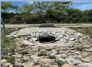
Culvert replacement on East Pekin Rd.
