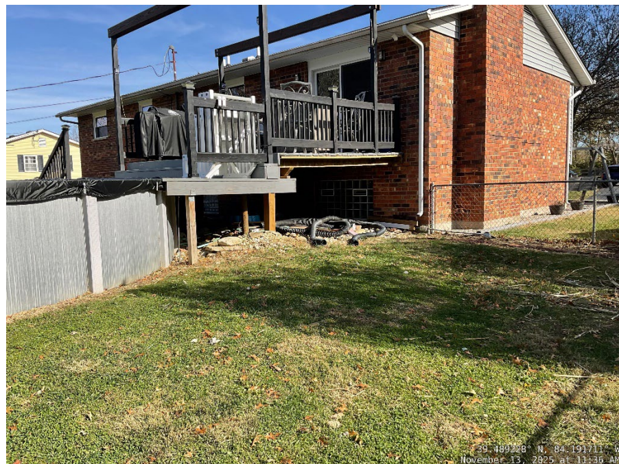
View looking northeast from southern property line.
