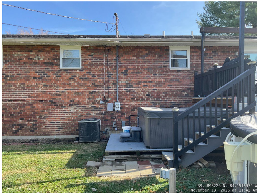
View looking east from septic tank lids.
