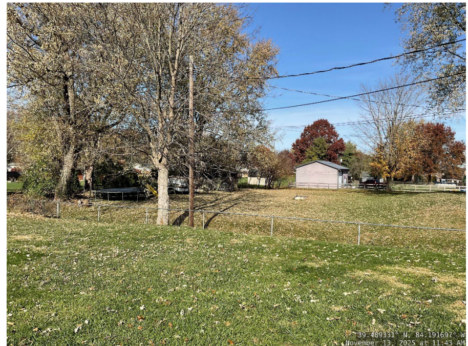
View looking northwest from septic tank lids.
