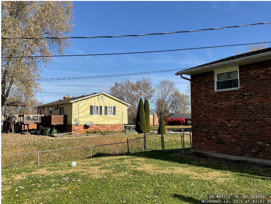
View looking northeast from septic tank lids.
