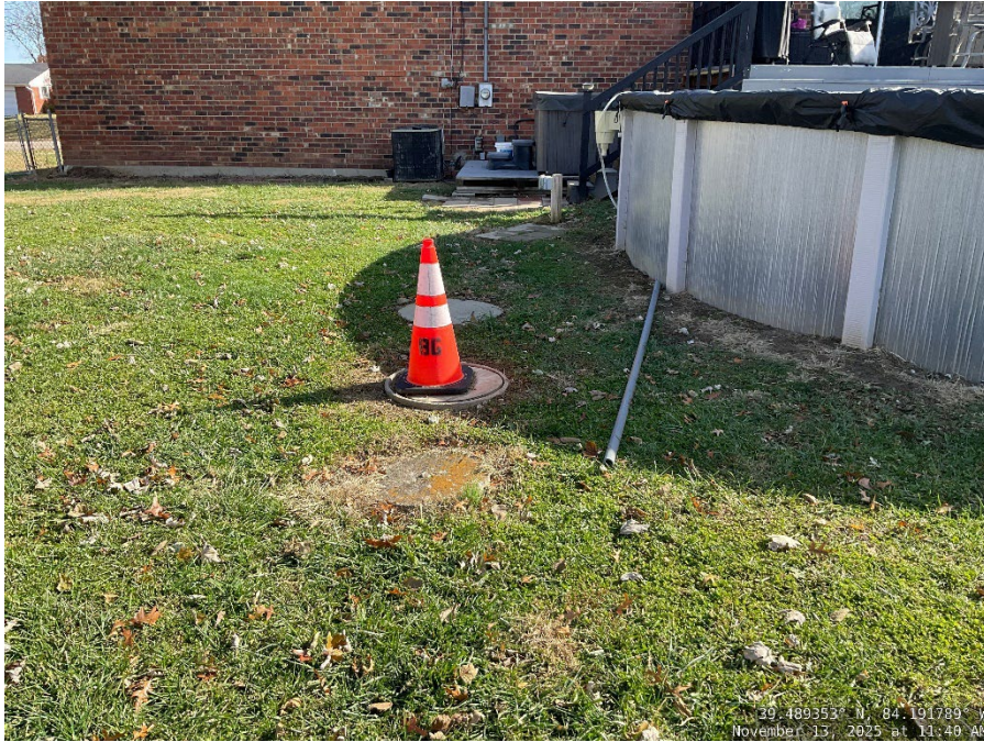
View looking east, note septic tank lids.
