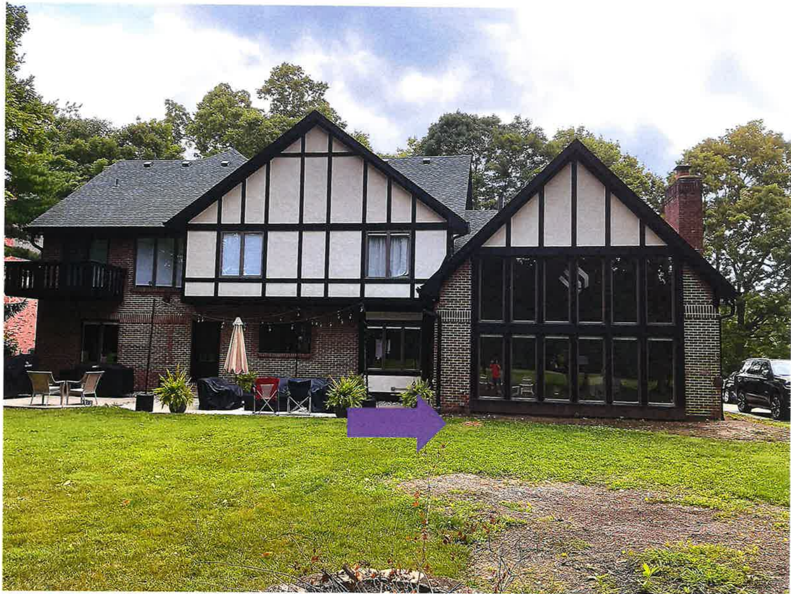
View looking at rear of house from the rear property line. Purple arrow identifies approximate western location of proposed addition.
